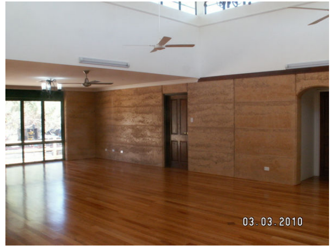
Internal Rammed Earth Walls
