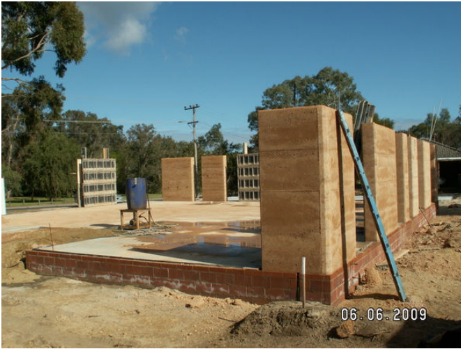
Rammed Earth Walls
